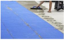
**8** Laying of the underlayment and decoupling mat BLANKE PERMAT with thin-bed mortar C2 S1 according to DIN 12004 or 12002.
