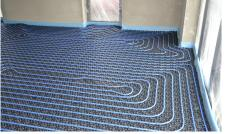
**5** Lay the BLANKE BF/C PIPE in the system in the specified spiral or serpentine pattern according to the plan and the surface heating and cooling system calculations, observing the recommended installation gap. The minimum installation gap is 10 cm, the maximum installation gap 25 cm. The minimum bending radiuses of  $16 \times 2$  mm and  $14 \times 2$  mm of the PE-RT heating pipe must not fall short of 8 cm (90° deflection) or 16 cm (180° deflection)
