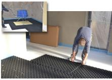
The system studded panels must be laid with an overlap of 50 mm. When overlapping at both sides, the studded panels can be clicked into each other.
