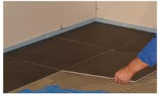
Daying of tiles on the underlayment. When laying BLANKE PERMAT and tiles, a thin-bed mortar C2 S1 to DIN 12004 or 12002 must be used. In the case of natural stone, an appropriate, suitable thin-bed mortar must be used.
