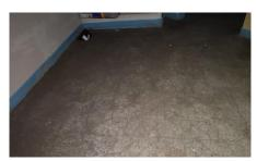
7 Once the thin layer of screed is applied (8 - 25 mm) and is ready to be walked on, it must be protected and shielded until the final floor covering is laid.
