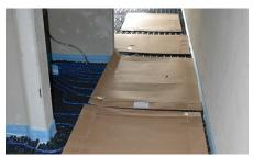
Please avoid any stresses such as walking on the system panels, positioning ladders or erecting scaffolding, or storing equipment and loads on them. If walk-ways are to be permanent fixtures, or equipment such as uncoilers need to be set up in the property, these areas must specially covered over and protected to ensure that the studs are not pressed in or damaged.
