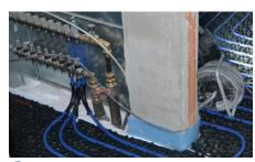
6 In the area of the heating circuit manifold, insert the BLANKE BENDS in order to achieve a clean connection and predefined 90° radius.
