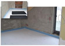
Affix system edge insulation strips to all vertical structural elements. Rest the base of the edge insulation strip on the top insulation layer or on the existing substrate. When using bonded fillers under the system studded panel, we recommend the installation of a protective, separating layer made of PE (polyethylene) with a thickness of at least 0.15 mm and with an overlap of 10 cm.
