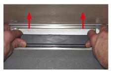
$2\,$  Grip the siphon on both sides and press it out of the drain connection; this is towards the wall or away from the wall depending on the installation situation.
