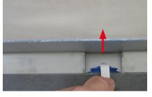
$2 \begin{array}{c} \text{Push the grate lifter up into the groove of the} \\ \text{drain connection nozzle and press it out; this} \\ \text{is towards the wall or away from the wall depending on the installation situation.} \end{array}$
