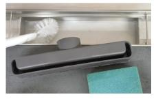
3 Remove coarse soiling in the channel body with flowing warm water and household cleaning products. A sponge or a brush is help-ful here. The same procedure has to be applied on the siphon. Grease the insertion connector of the siphon prior to reinstillation (e.g. with fitting grease or Vaseline).
