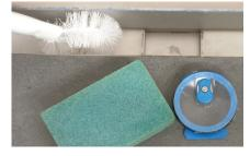
**3** Remove coarse soiling in the channel body with flowing warm water and household cleaning products. A sponge or a brush is helpful here. The same procedure has to be applied on the drain connection nozzle. Grease the sealing ring of the drain connection nozzle prior to reinstillation (e.g. with fitting grease or Vaseline).
