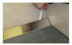
**1** The grate cover is raised and lifted out using the grate lifter (white plastic lever) included in the scope of delivery.
