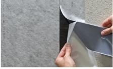
As a last component, apply the BLANKE DISK AB edge tape to the remaining fleece-free overlap areas of the waterproofing membrane. Here too, uncover 5 cm of the plastic cover, apply the edge tape and press it against the wall by hand to eliminate bubbles while removing the plastic cover on the rear.
