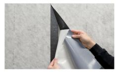
6 Affix additional waterproofing membranes to the fleece-free areas of the BLANKE DISK waterproofing membrane, and press them firmly into place by hand ensuring that bubbles are removed. Use a cutter knife to cut BLANKE DISK to size.
