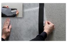
5 Surface sealing is carried out using BLANKE DISK waterproofing membrane. Pull off roughly 5 cm of the plastic cover on the reverse of the narrow part, apply the strip to the substrate and gradually press it against the surface to eliminate bubbles when removing the plastic cover on the reverse.
