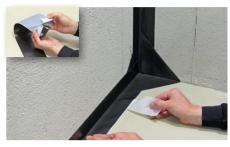
**3** Fit BLANKE DISK TAPE to all horizontal and vertical corner areas. Pull off roughly 5 cm of the plastic cover on the reverse, apply the corner waterproofing membrane to the substrate and press it against the surface to eliminate bubbles while removing the plastic cover on the reverse. Overlap the products by 5 cm.
