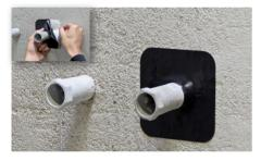
4 Pipe openings must also be sealed with BLANKE DISK WM/BM wall and floor collars before applying the waterproofing membrane. Ensure that the sealing collar forms a proper collar at the pipe extension required.
