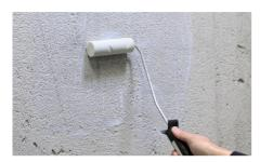
All substrates must be dry, capable of bearing the load and free of any layers that could impair bonding. The flatness specification must meet DIN 18202 requirements. Apply primer coating BLANKE GROUND to wall and floor surfaces according to their surface condition. Observe the specified drying time.
