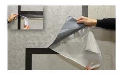
In order to use leftover pieces of BLANKE DISK waterproofing membrane on the surface, apply BLANKE DISK TAPE at a 90° angle to the existing waterproofing membrane on the fleece-free area. Then align the joint area of the two waterproofing membranes with an overlap of at least 5 cm on the BLANKE DISK TAPE.
