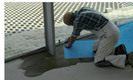
4. The mats have a glass fibre mesh overhang of approx. 3 cm (1") on two adjoining sides. These overhangs are needed to join the mats at their seams. It is not necessary to further reinforce the joints of the mats. Abut the mats tight to each other and avoid any gaps between them.
