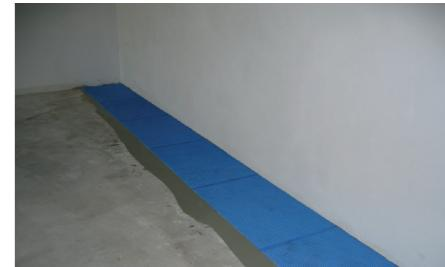
1. Substrates must be clean, load bearing, and free from non-adherent substances. The flatness must correspond to DIN 18202. If necessary, apply a primer in accordance with the substrate.
