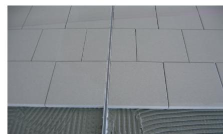
7. Fill the cavities of the glass grid structure evenly with thin-set mortar. Then apply sufficient mortar to the area, wet-on-wet, then comb using a notched trowel appropriate for the tile or stone installation. Embed the tiles in thinset.
